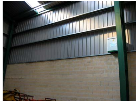
Figure #9: High-located equipment to ensure proper protection from contacts.
