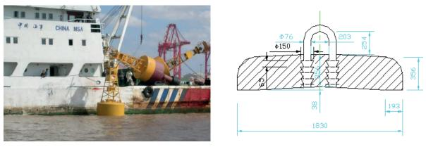
Figure 7 : Installation of light buoy
