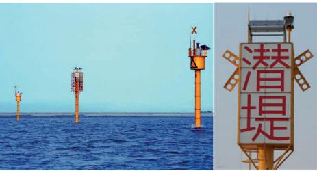
Figure 5: Installation of warning signs in guiding dikes
