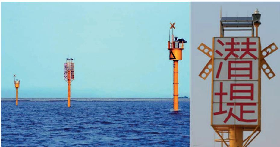
*Figure 5: Installation of warning signs in guiding dikes*
