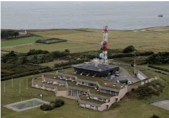
CROSS Corsen (1982) at Corsen Point (Brittany - France)
