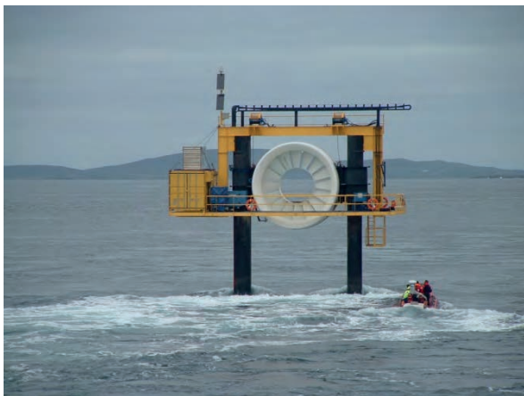
OpenHydro pile-mounted turbine at EMEC tidal test site
