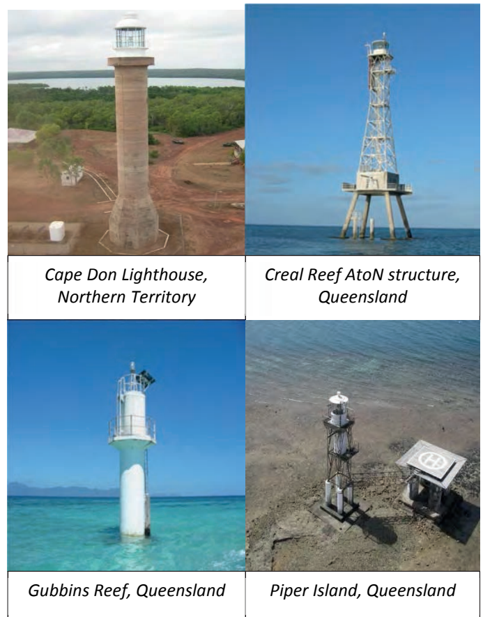
Figure 2: Photos of AtoN structures with concrete materials
