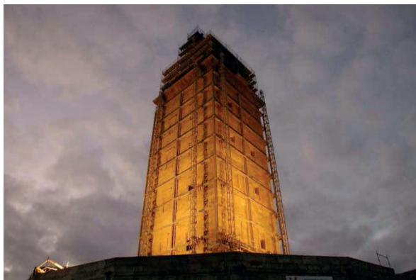
Image 8: Building works in the Tower of Hercules 2009
