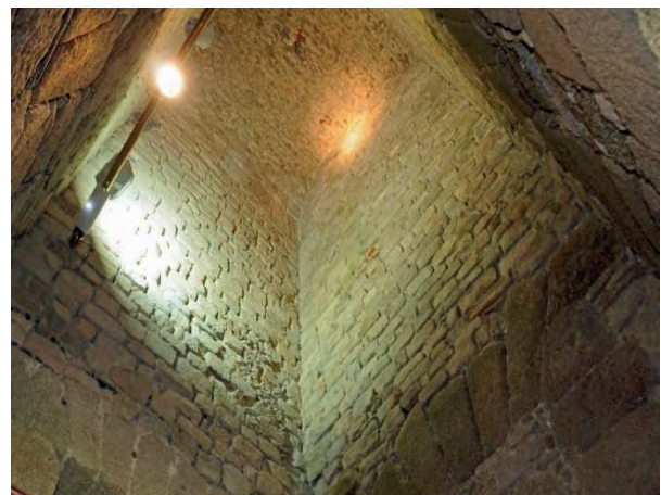
Image 4: Roman constructive systems in chambers of the internal nucleus of the Tower
