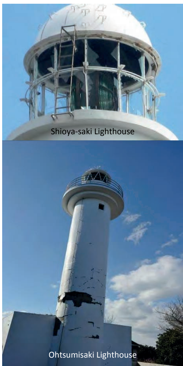
Figure 5: Examples of damage (broken lantern panels and cracked lighthouse)
