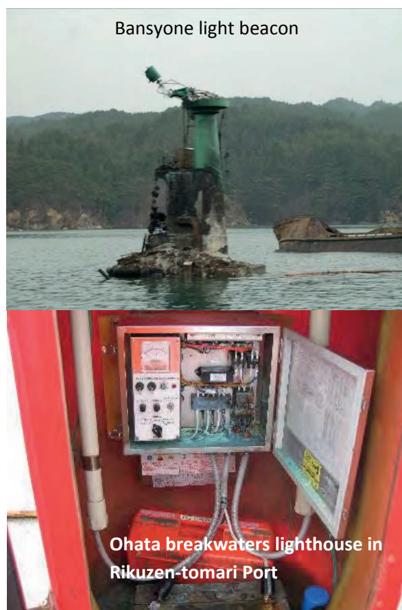
Figure 4: Examples of damage (burned out and submerged AtoN)
