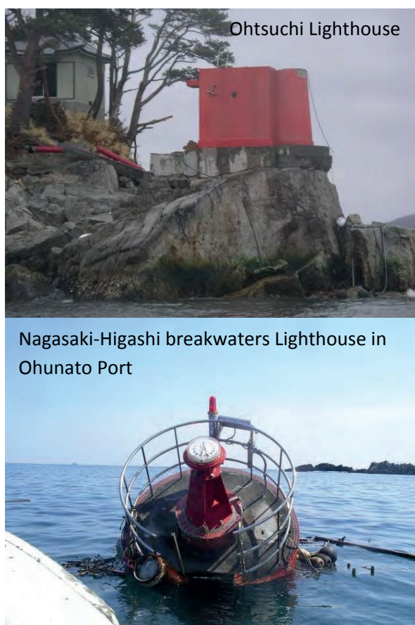
Figure 3: Examples of damage (collapsed and tilted lighthouses)
