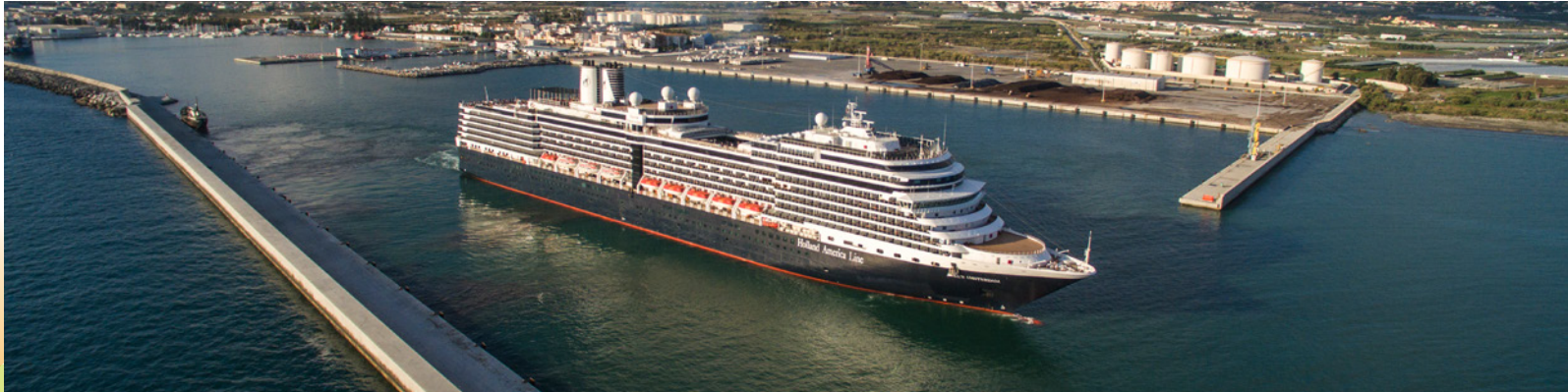
Vista general del muelle Dique. / General view of the Dike dock.
