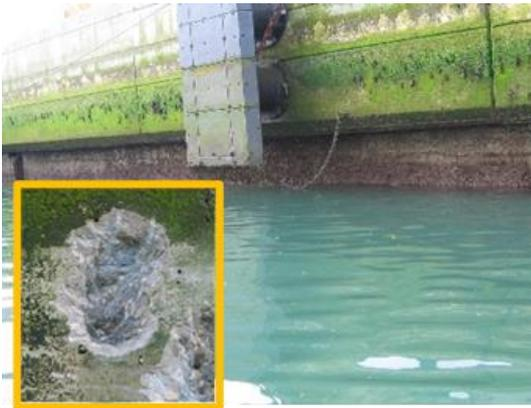
Photograph 13. Dock made with floating caissons in an XS3 environment, 2 years of service. Close-up of bars uncovered, with no signs of corrosion. BFS cement, 32,5-SR
