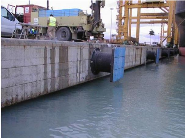
Photograph 16 Extraction of specimens in Valencia Port
