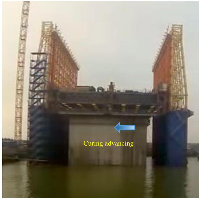
Photograph 8. Example of the curing process during the construction of caisson on a floating platform [17]
