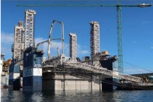
Photograph 1. floating platform with a caisson in construction, partially submerged
