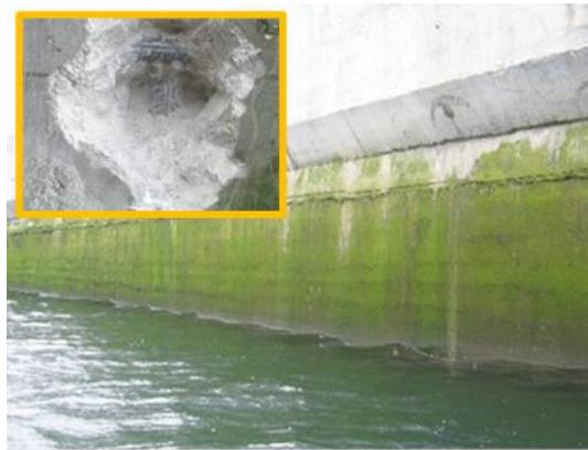
Photograph 14. Dock made with floating caissons in an XS3 environment, 2 years of service. Close-up of bars uncovered, with no signs of corrosion. Pozzolanic cement, 32,5-SR/MR
