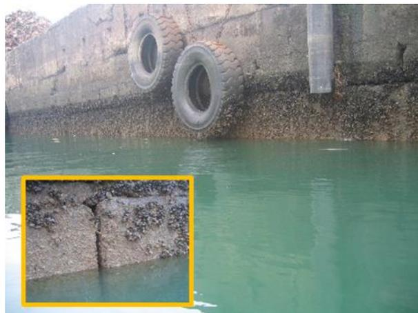
Photograph 15. Dock made with floating caissons in an XS3 environment, 31 years of service. Without signs of corrosion. Pozzolanic cement
