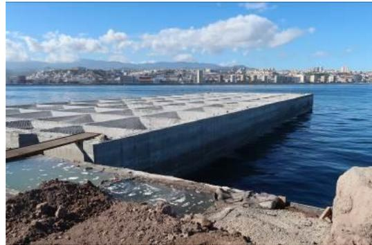
Photograph 2. Caisson at the final location in the breakwater
