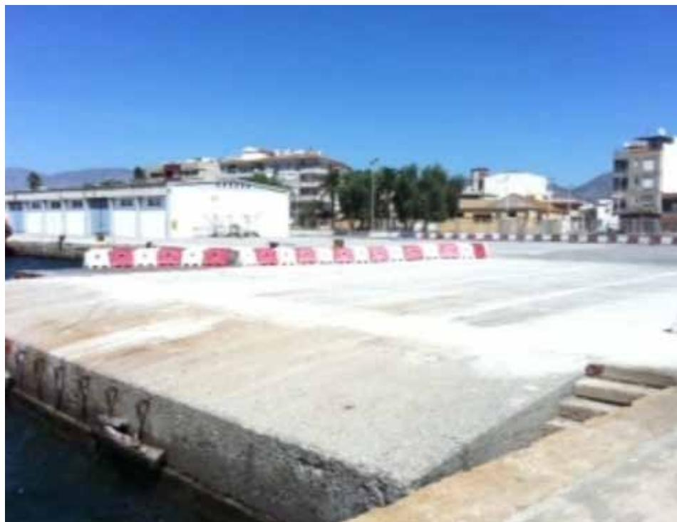
In order for ships docked at the West Dock to be able to function and operate efficiently, it was necessary to remodel the RORO ramp. Work essentially consisted of removing a mooring bollard and refurbishing the floor of the ramp and its access road.
