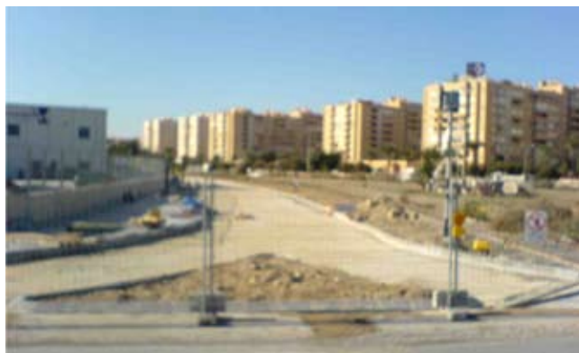
Entronque vial acceso al contradique con vial existente. Y Junction on access road to counterdyke with existing road.
